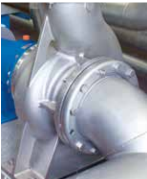
Highly efficient stainless steel centrifugal pump
